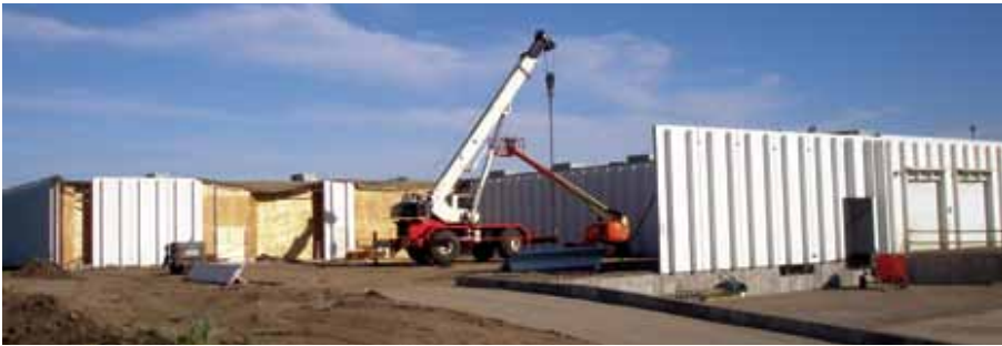
WSI relocate wall panels for building addition.
